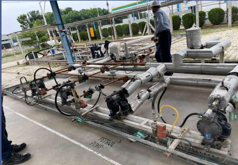
Diaphragm Pumping Station
