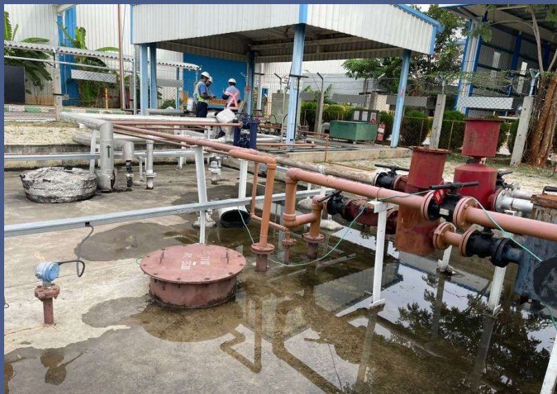
Underground Petrol Tanks
